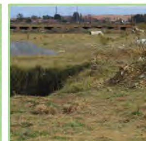
Picture 31: Exposed excavation
