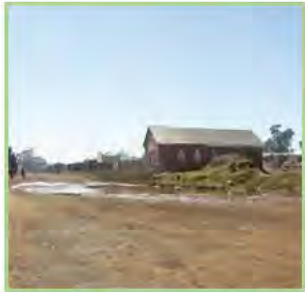
Picture 33: Ponding water on gravel road
