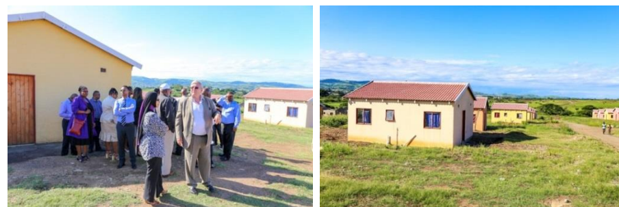
The multi-year housing project seeks to construct approximately 3 000 houses.
