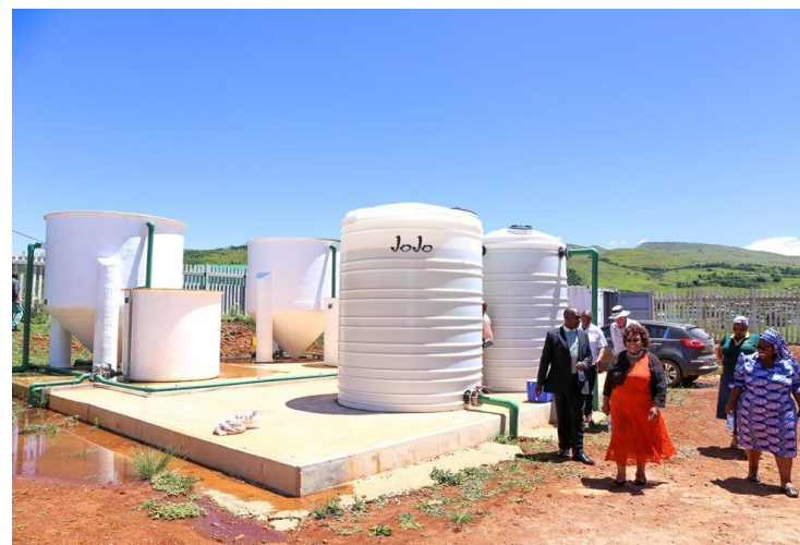
The water treatment works facility in Impendle.
