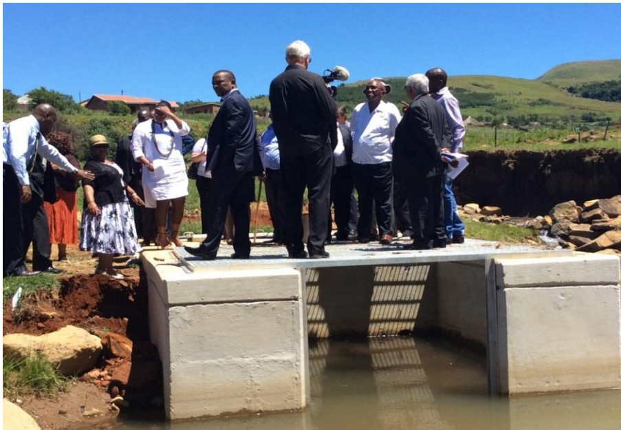
The river where the water distribution facility was constructed for supplying the reservoir – previously, communities had to fetch their daily water with buckets.
