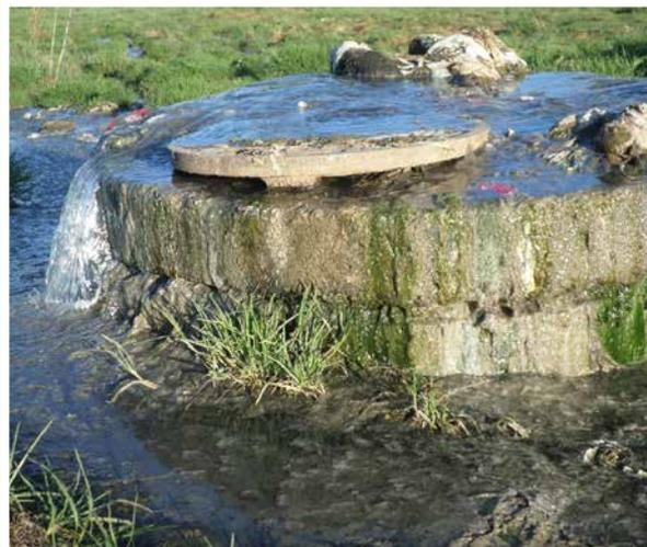
*Phuthadijhaba wastewater treatment works is non-functional due to serious vandalism, resulting in sewage overflows in the area (Maluti-A-Phofung, Free State)*
