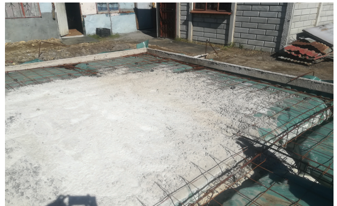
Incomplete concrete slab and foundation
