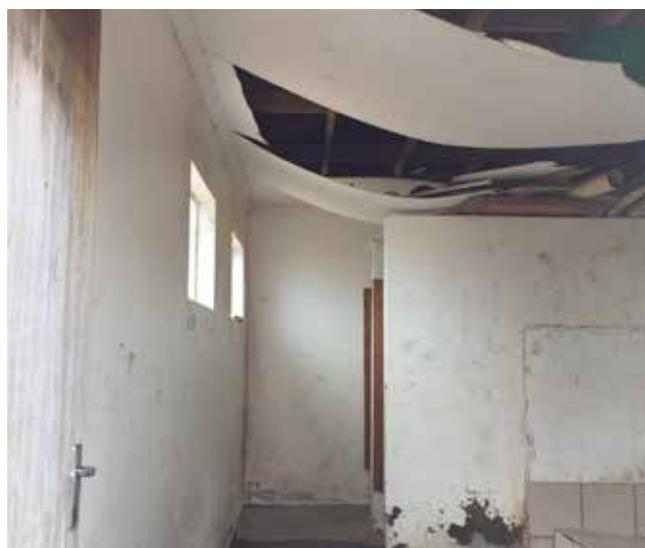
*Blocked toilets and ceiling close to collapsing*
