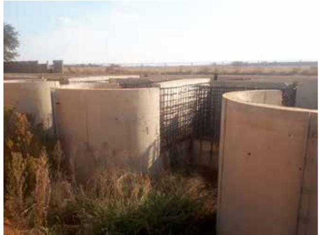
*Reinforcing steel severely affected by rust*
