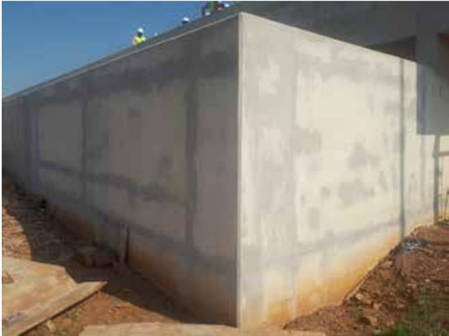
*Lots of patched cracks on concrete*
