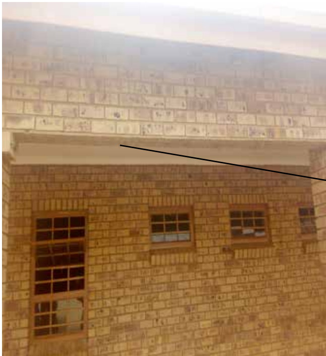
Bricks fallen from edge arch
