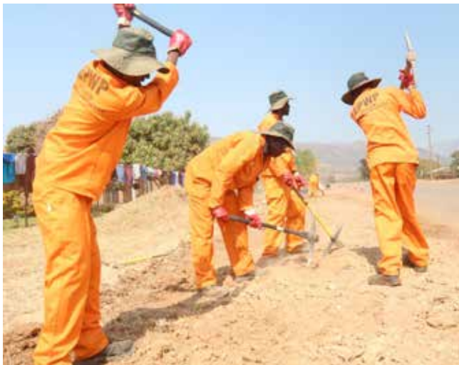
EPWP workers on site
