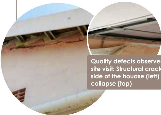
Quality defects observed during site visit: Structural crack on the side of the house (left) and ceiling collapse (top)
