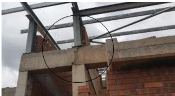
Concrete beams cast separately in parts, with visible cracks and concrete overlap in attempt to repair cracks
