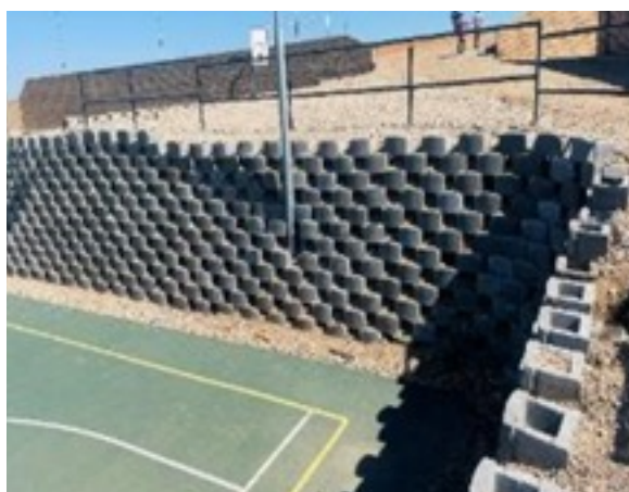
Top retaining wall blocks loose
