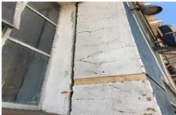
Police station – cracked column
