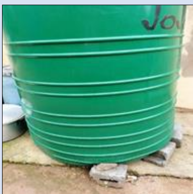
Tank missing a tap and placed on loose concrete brick (left); unused tank placed on uneven ground (right)
