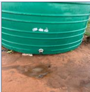
Water tank outlets with inadequate ground clearance (left) and stagnant water around water tank with tank outlet broken (right)
