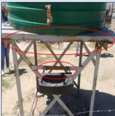
Visible signs of corrosion of the steel stand for the water tanks (left) and poor concrete foundations (right)
