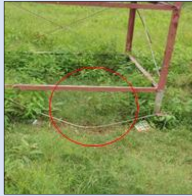
Overhanging water tank on a steel structure of smaller dimension than tank (left) and cross braces that were damaged and loose, weakening the steel structure (right)
