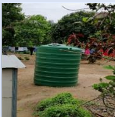
Tank missing a tap and placed on loose concrete brick (left); unused tank placed on uneven ground (right)
