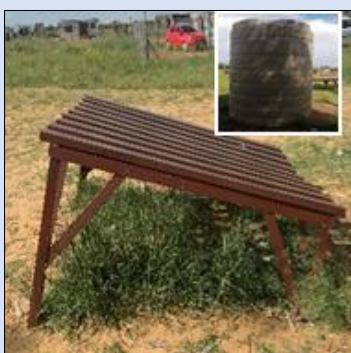
Water tank structures were not level (left and right); Water tanks stored directly on ground with no stands due uneven water tank structures (inset)
