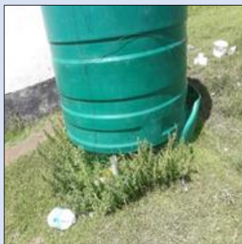
Water tanks placed on uneven surfaces and supported by loose concrete blocks
