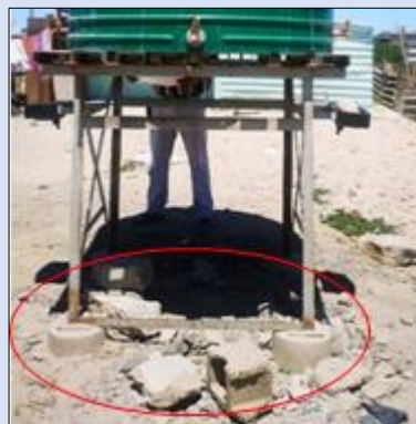
Visible signs of corrosion of the steel stand for the water tanks (left) and poor concrete foundations (right)
