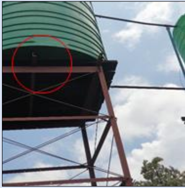
Overhanging water tank on a steel structure of smaller dimension than tank (left) and cross braces that were damaged and loose, weakening the steel structure (right)
