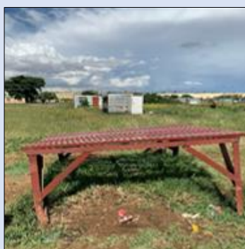
Water tank structures were not level (left and right); Water tanks stored directly on ground with no stands due uneven water tank structures (inset)
