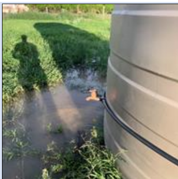
Water tank outlets with inadequate ground clearance (left) and stagnant water around water tank with tank outlet broken (right)
