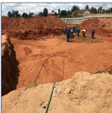
Moshate project: Project was incomplete on 10 December 2020, with contractor still on earthworks in preparation for the foundation for steel tank base
